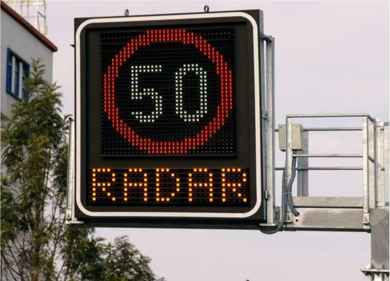
This smart road sign receives data and modifications to better inform drivers and prevent congestion or accidents.
